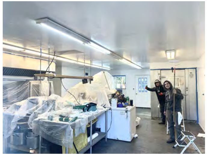
Sprucing up the kitchen with fresh paint
