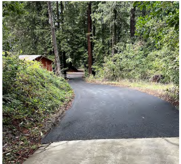
Newly-paved upper portion of stupa access road
