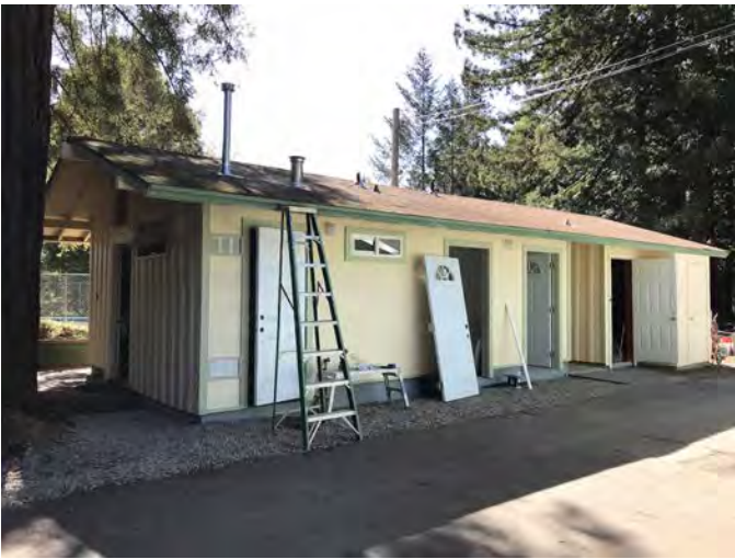
Accessible bath house at the pool and dining hall
