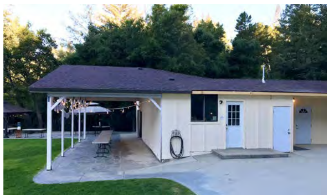
Meadow annex serving area roof
