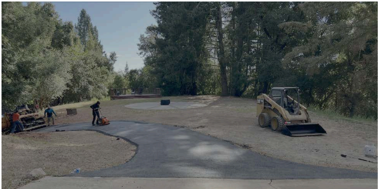
Paving the Eastern Cabin Road
